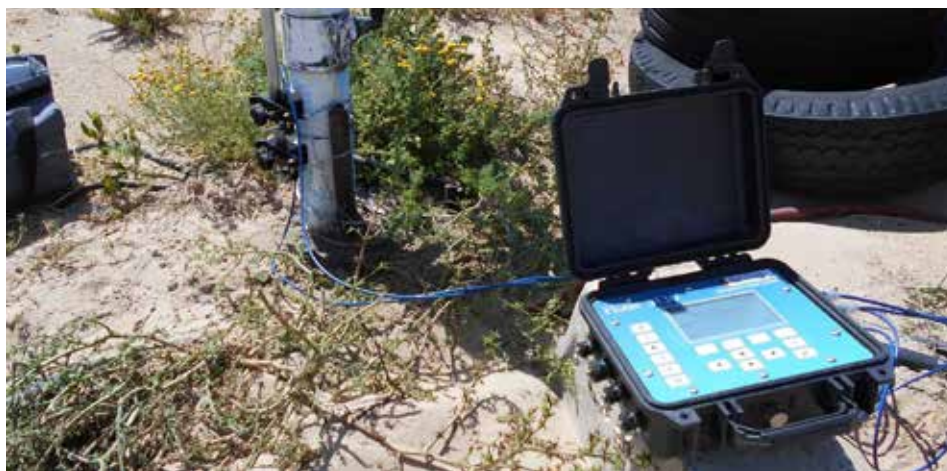
Figure 6: Using a portable flow meter to determine the water flow rate of a centre pivot irrigation system
